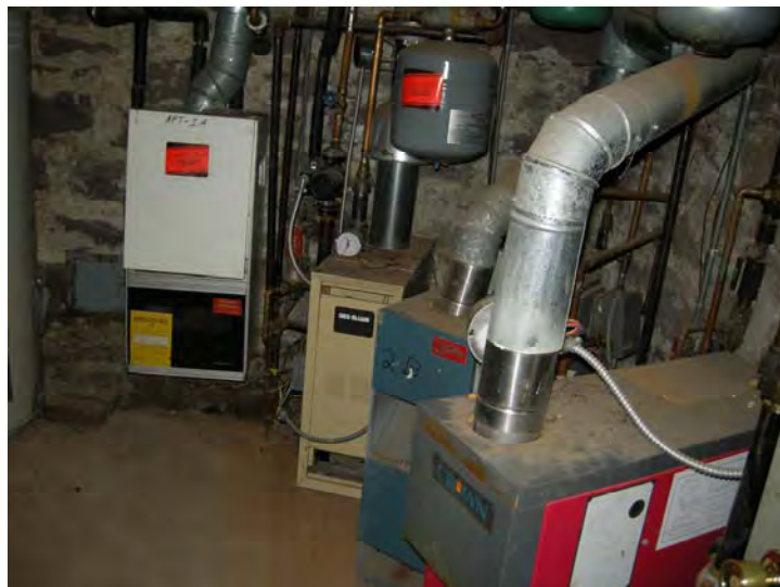
Typical array of standard floor mount and wall mounted heating boilers
