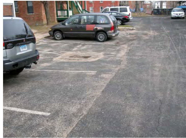
The sunken storm drain at 42-48 Wolcott
