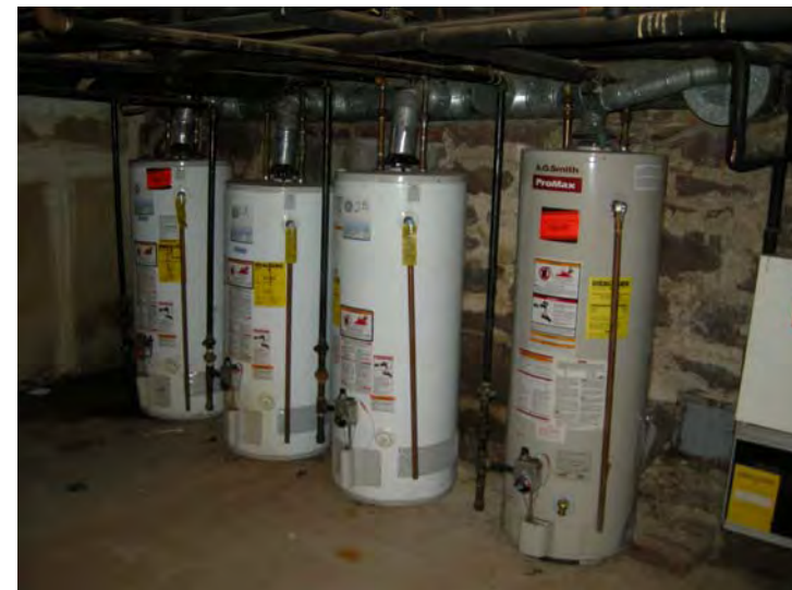
Typical array of domestic hot water heaters.
